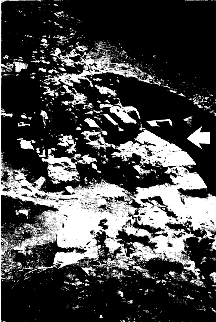
Fig. 3. Deformation of the southern wall of the Ateret Fortress looking east. Arrow points at fault zone. Location is shown in Fig. 2.
